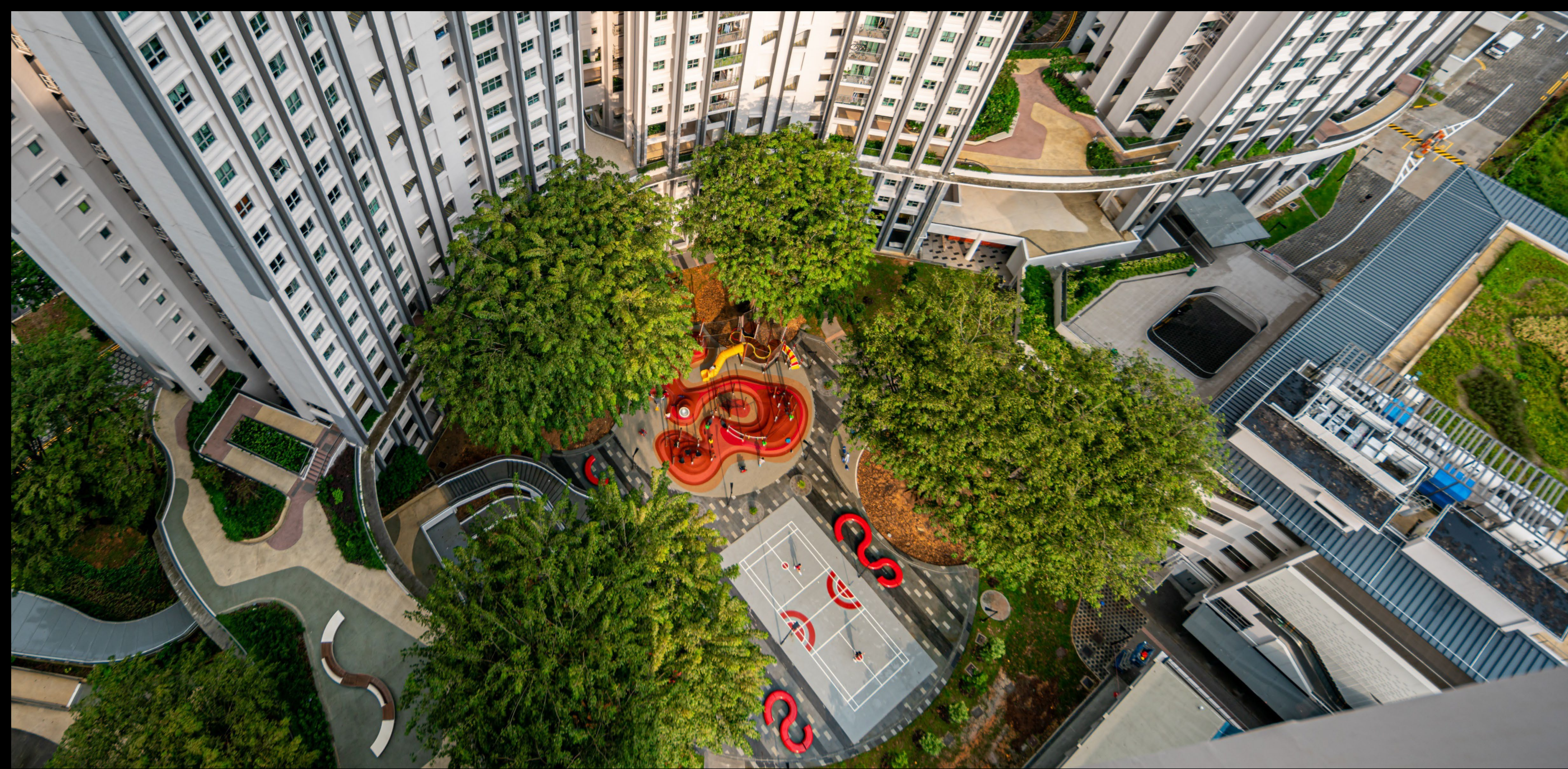
The Central Plaza is designed to re-create the old town square, injecting vibrancy into the precinct and surrounded by residential blocks and amenities
