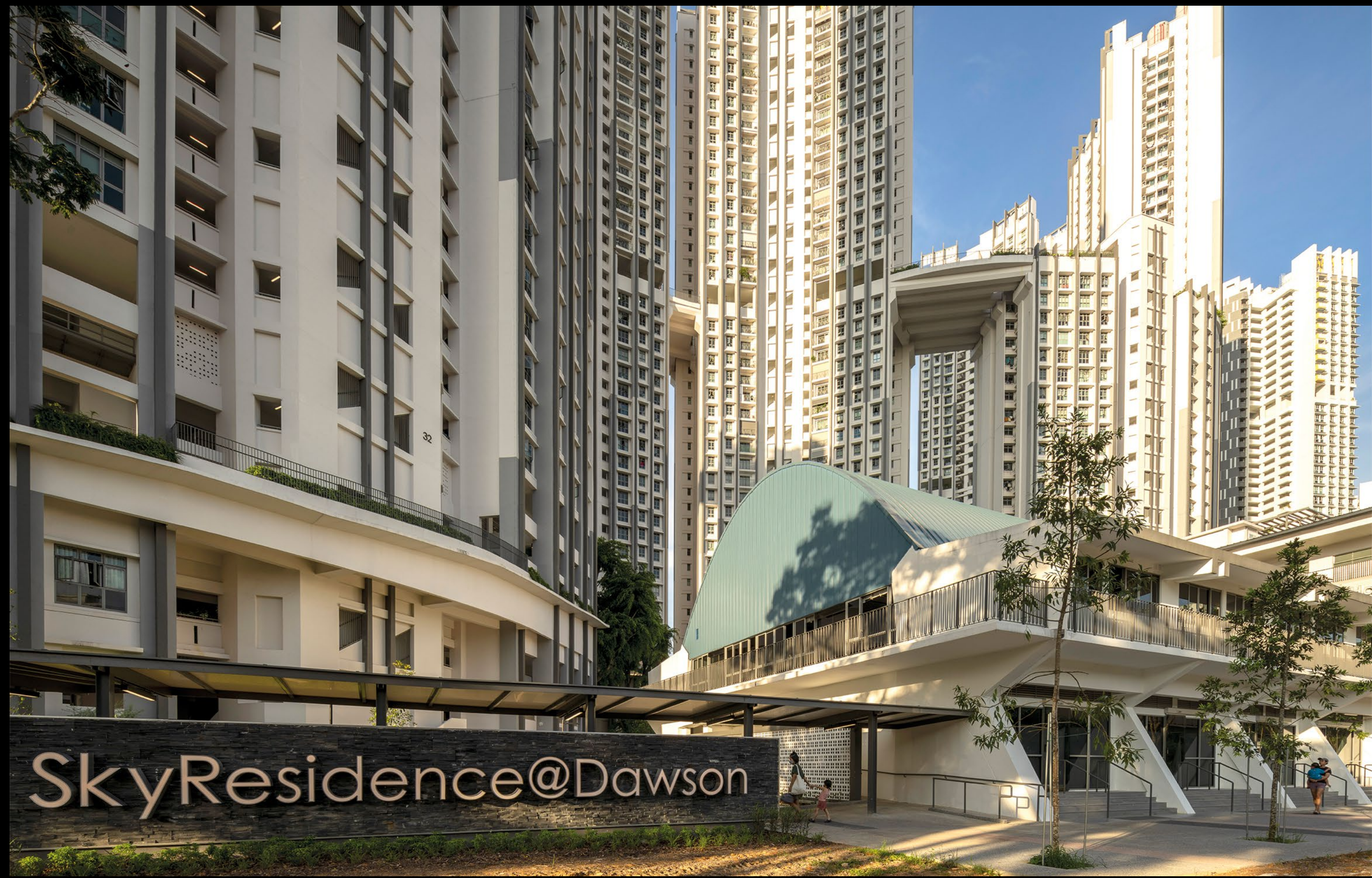
The former wet market building was revitalized to retain its old charm, creating a lifestyle destination for residents
